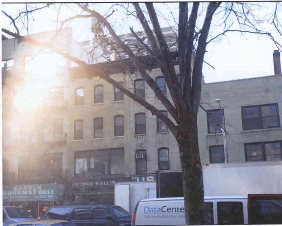
View of the west side of 6 th Avenue from 800 6 th Avenue looking west.
