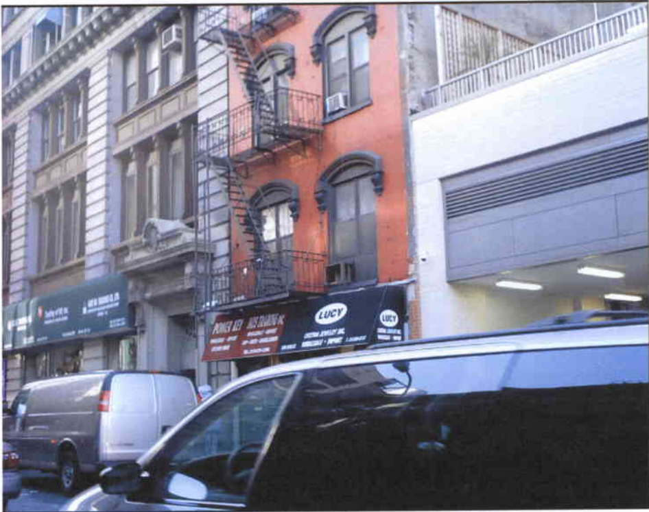
View of the adjoining properties to the west of the project site from 6 th Avenue.
