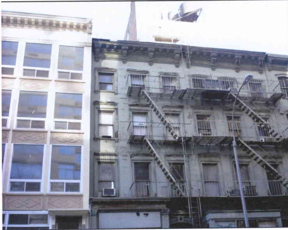
View across West 28 th Street looking north-northeast from the project site.
